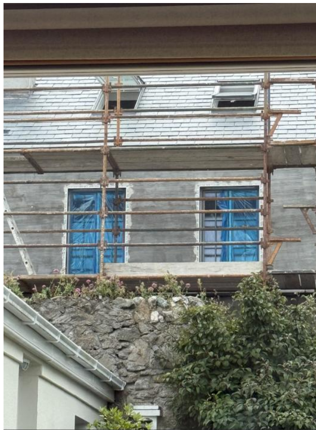
Figure 4 - Photo showing direct sightline from rooflights to living room sofa
