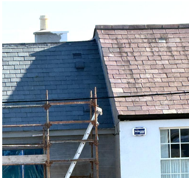
Figure 5 - Photo showing neighbouring elevation (no. 6 Sorrento on right)
